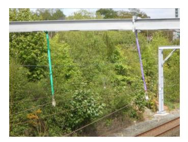
At Eccles the wiring seems to have got ahead of the provision of insulators and supports, so in a number of places it is hung temporarily on nylon straps with pulleys.
