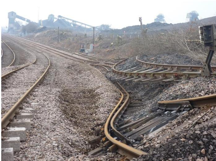
*The twisted track at Hatfield Colliery, as a result of the landslide.*
