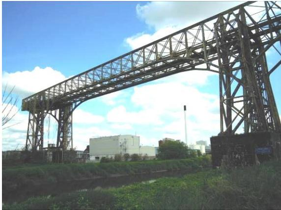
Pictured on the 18<sup>th</sup> June is the **railway transporter bridge** over the Mersey at Warrington. A branch line from Arpley yard goes under the main line south of Bank Quay station, but no longer links to the bridge.
