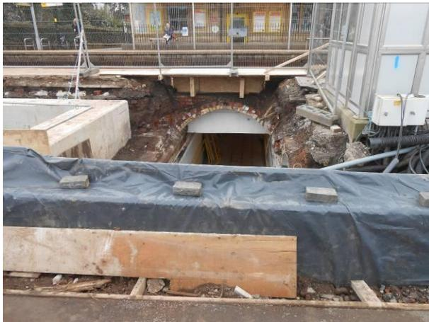
Here is the old underpass. It will be brought back into use with lift access for all four platforms.
