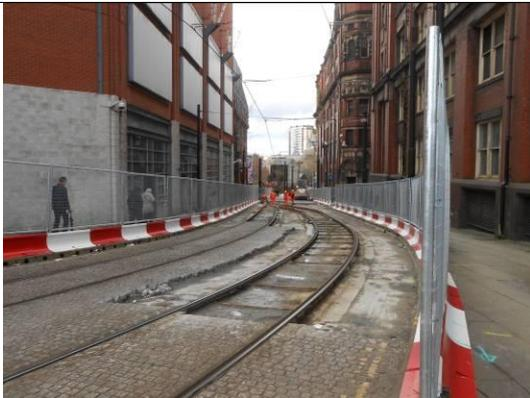
*While **Victoria tram stop is closed** for reconstruction the trams are operating on a **single line**. This has necessitated a point being placed just on Balloon Street between Shude Hill and Victoria.*
